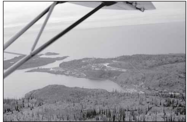
Aerial view of Eldorado Mining and Refining minesite, Port Radium Credit: Busse / NWT Archives / N-1979-052-3338
