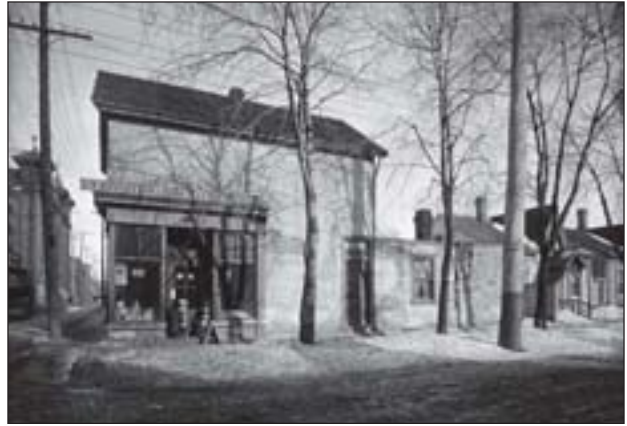
William Street (St. Patrick Street) and corner of Anderson Street (Dundas Street ~ Anderson Street widening), March 5, 1912
